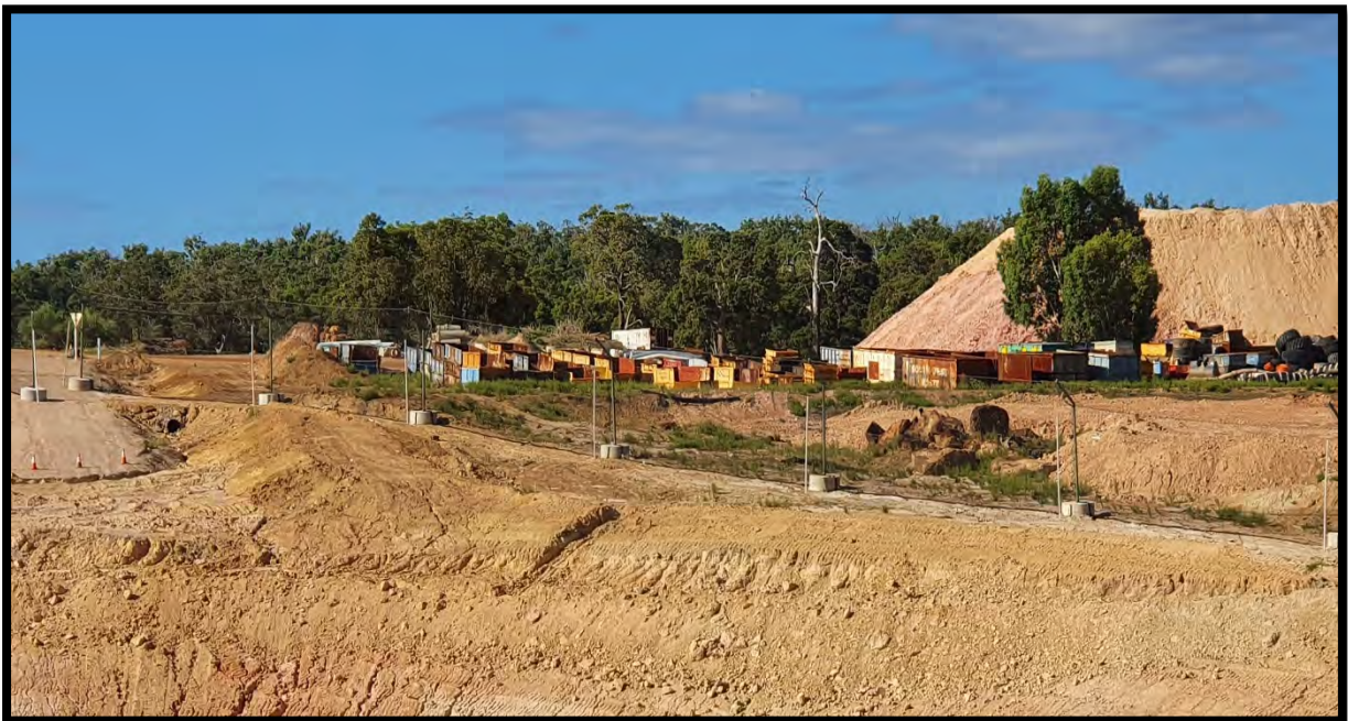
Plate 2. Cyclone fencing on the periphery of a waste cell.
