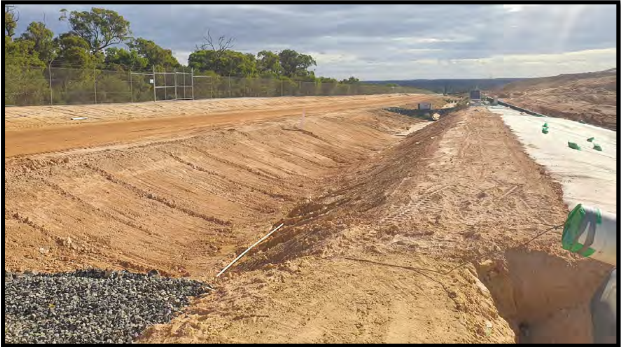
Plate 1. Cyclone fencing on southern property boundary and upgraded stormwater infrastructure.
